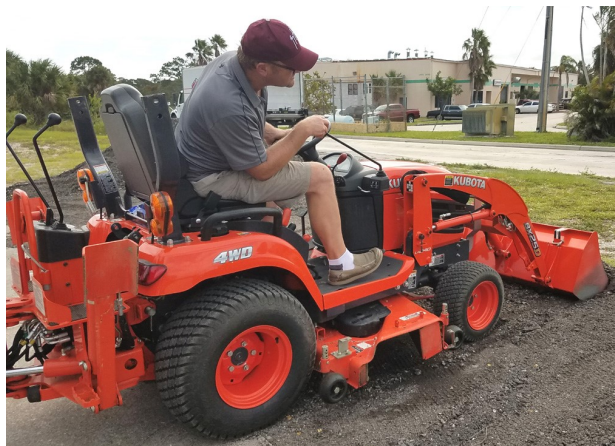
Parking Lot Improvement! Thanks Randy for donating your Kubota tractor and spreading asphalt in the VFW parking lot.
